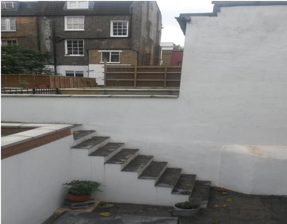
Photo 6: View of the existing basement lightwell to adjoining neighbour No.354 Caledonian Road and the extent of the two storey full width rear extension at No.352.
