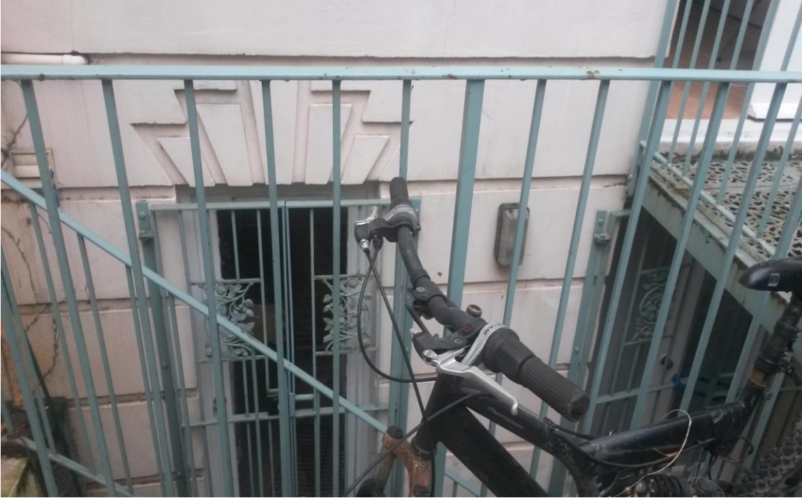
Photo 3: View of the existing rear lightwell.
